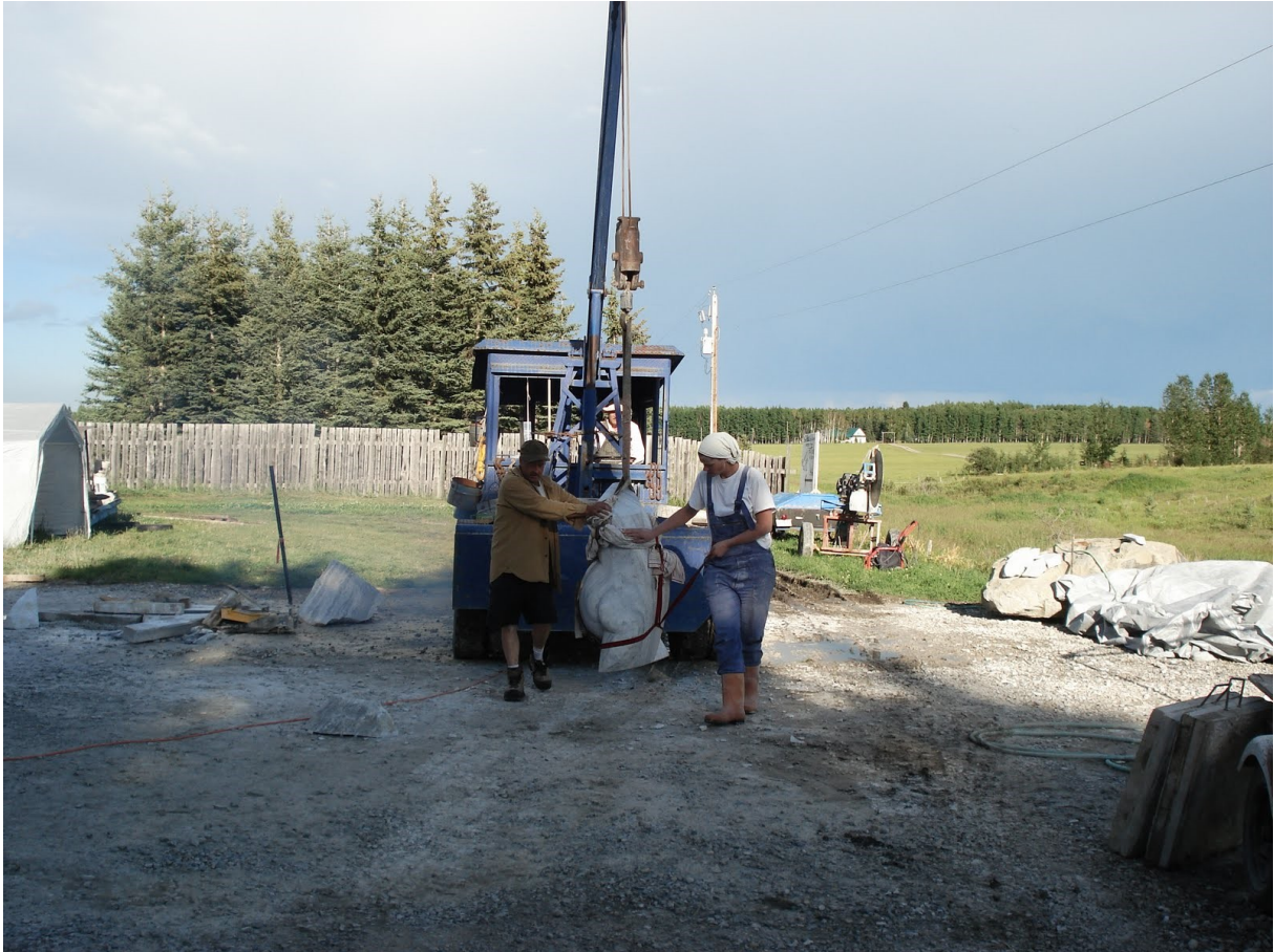
When it was time to install "Reflection" we used Old Blue to take the torso, the big crane took the base which wighs about 12,000lb I think.
